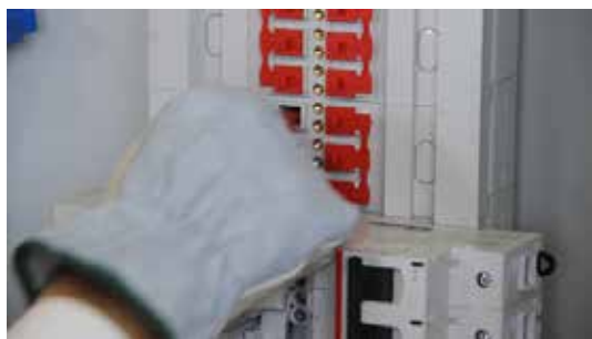
The Protective Cover Is Removed
