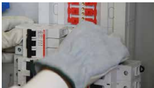
The Breaker Snaps Into The DIN Rail
