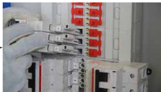
The Breaker Is Inserted Into The Opening
